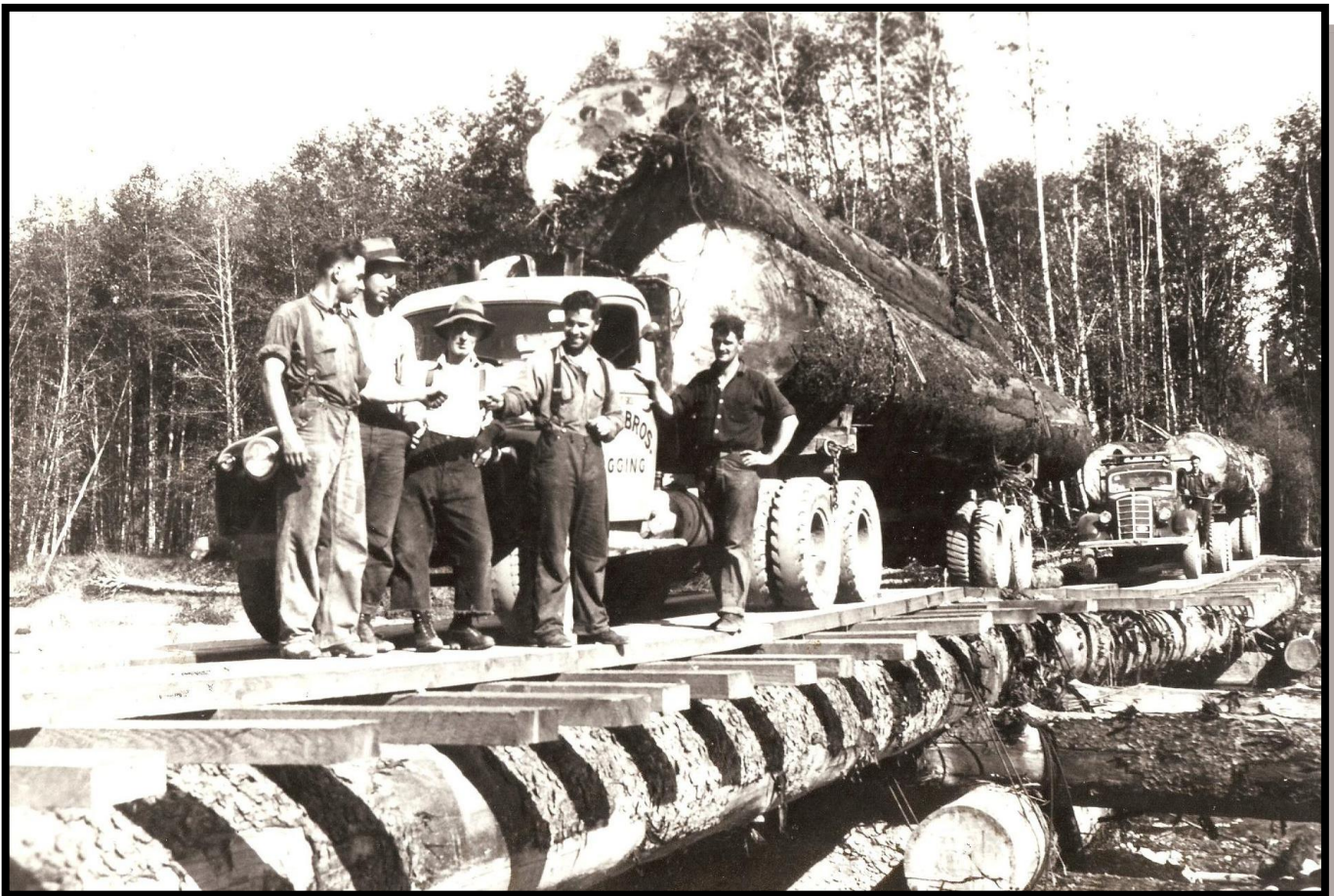
First loads across this bridge: "Bridge over the Queets River above the cable foot bridge and just above the mouth of Salmon River." Summer, 1943.
